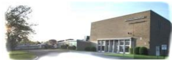
Figure 4: Greece Olympia School Campus
