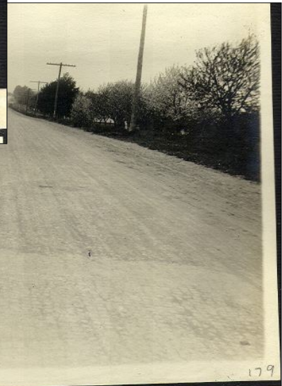
179. Cement cube pavement on Ridge road, Greece, looking to Hoosick Hill. 1909.
