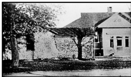
Stone Schoolhouse before demolition
